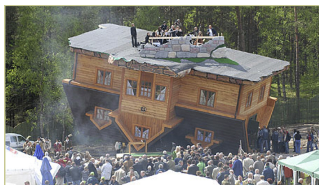
Fig. 2 – The Upside Down House in Szymbork. Source: www.szarlota.pl .
